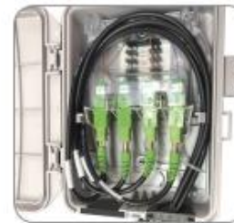
Clean and install premise drop connector
